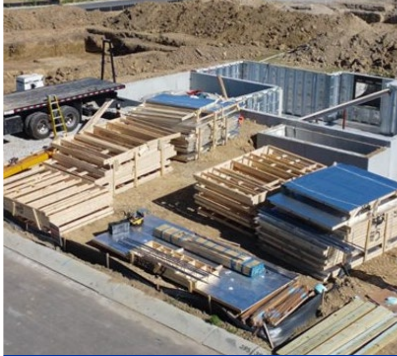
Staged floor trusses and wall panels for efficient on-site building.
